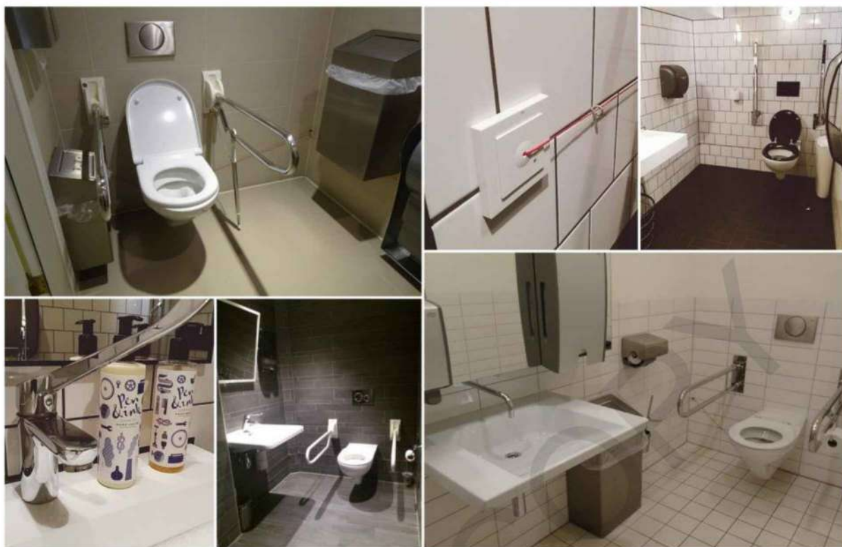
Figure 46: Example of lever type tap, foldable grab bars, etc. in accessible toilet type A (Source: https://www.ableamsterdam.com/wp-content/uploads/2019/06/accessible-toilets-2-1024x662.jpg )
