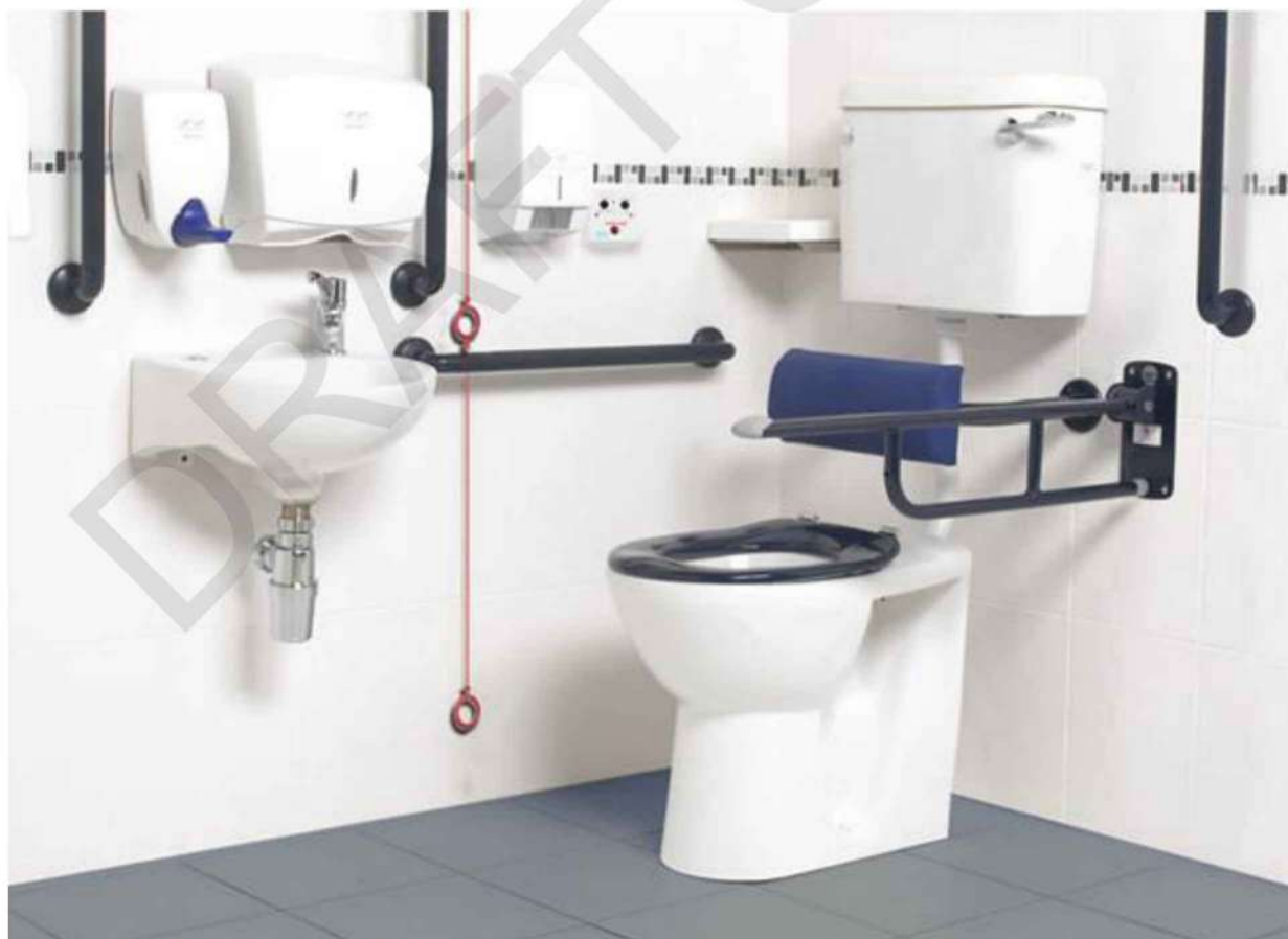
Figure 47: Example of type B toilet with emergency alarm pull chord at two levels (Source: https://www.disabilityaids.co.nz/wp-content/uploads/WC-Suites.jpg )
